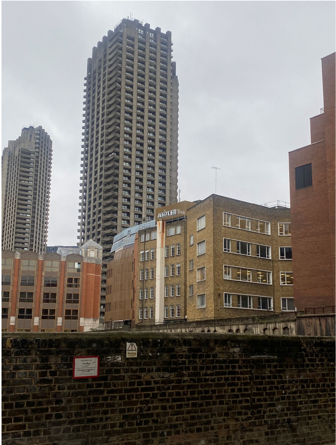
Image 7: The north of the site, alongside adjacent buildings, viewed from Hayne Street
